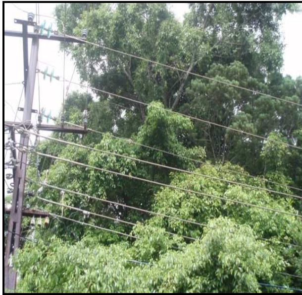
Figure 52: Vegetation growing into HV and LV lines
