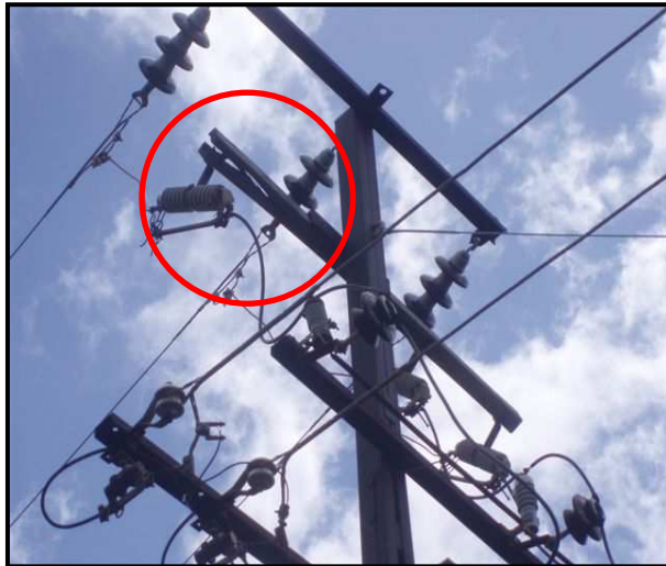
Figure 54: Example of failed cross-arm in Darwin Network
