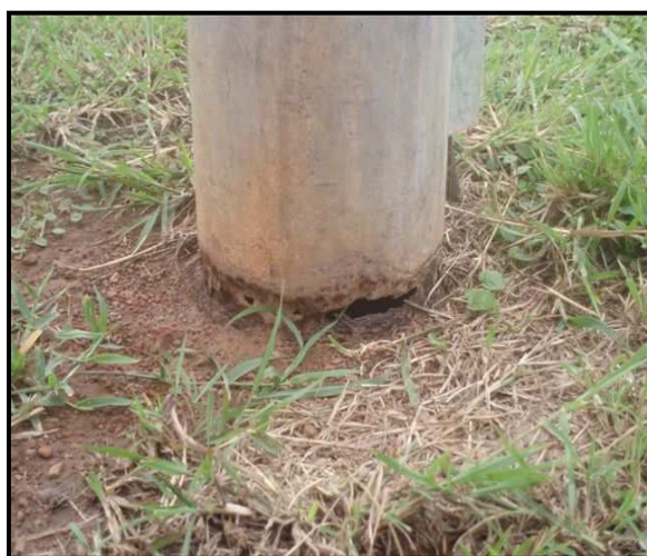
Figure 51: Rust affected steel street light pole in Darwin Network
